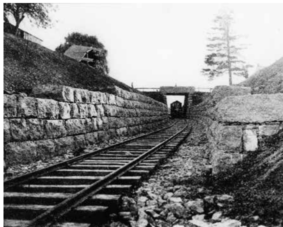
Northbound steam train passing through the new Hurley cut, 1903, HHS Collection. Notice barn cut in half at upper left to make room for the railway construction.
